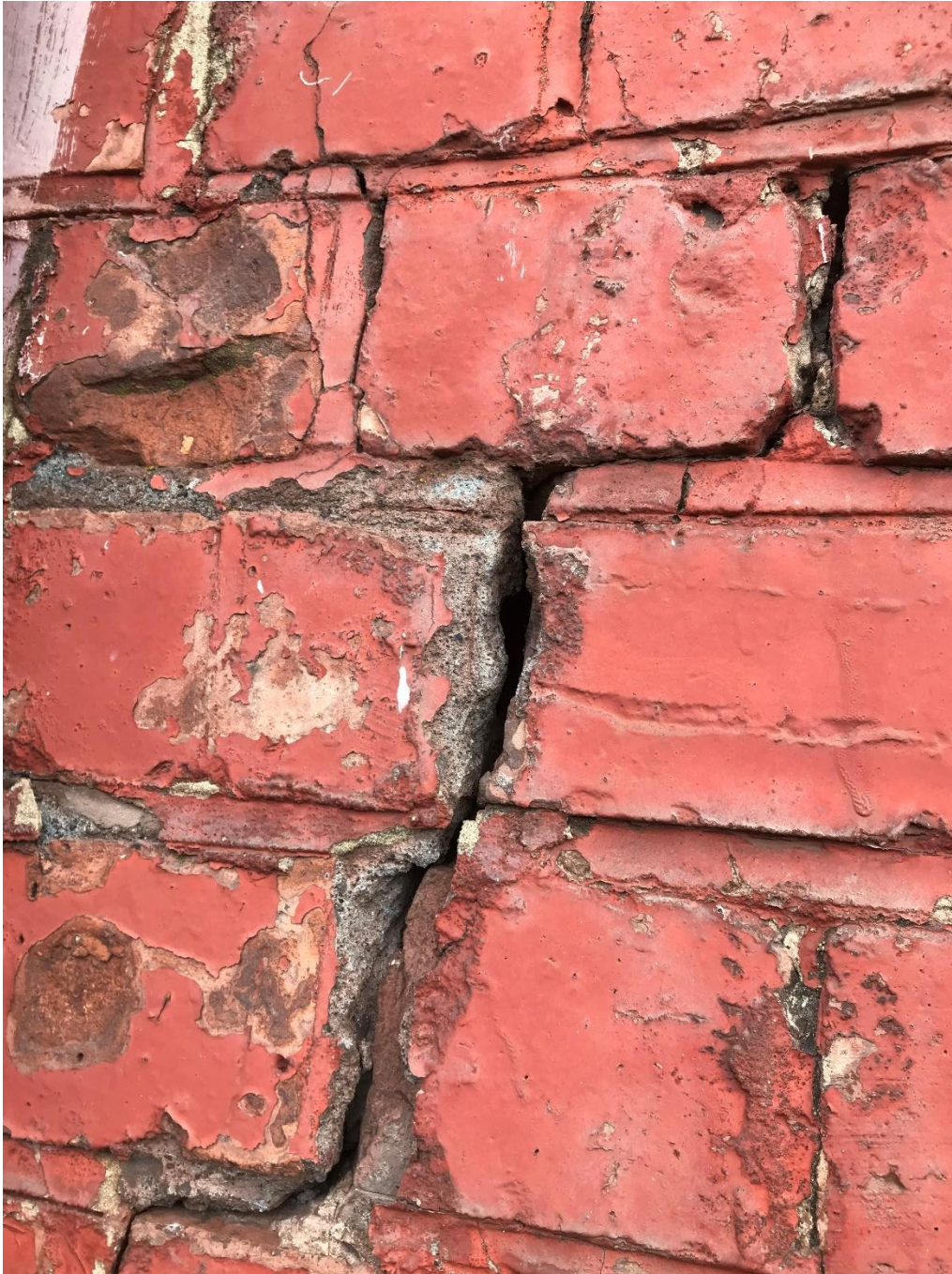
Photograph 8 – Subsidence crack in southern-western wall of structure B1b, potentially leads to wall cavity but cobwebs inside
