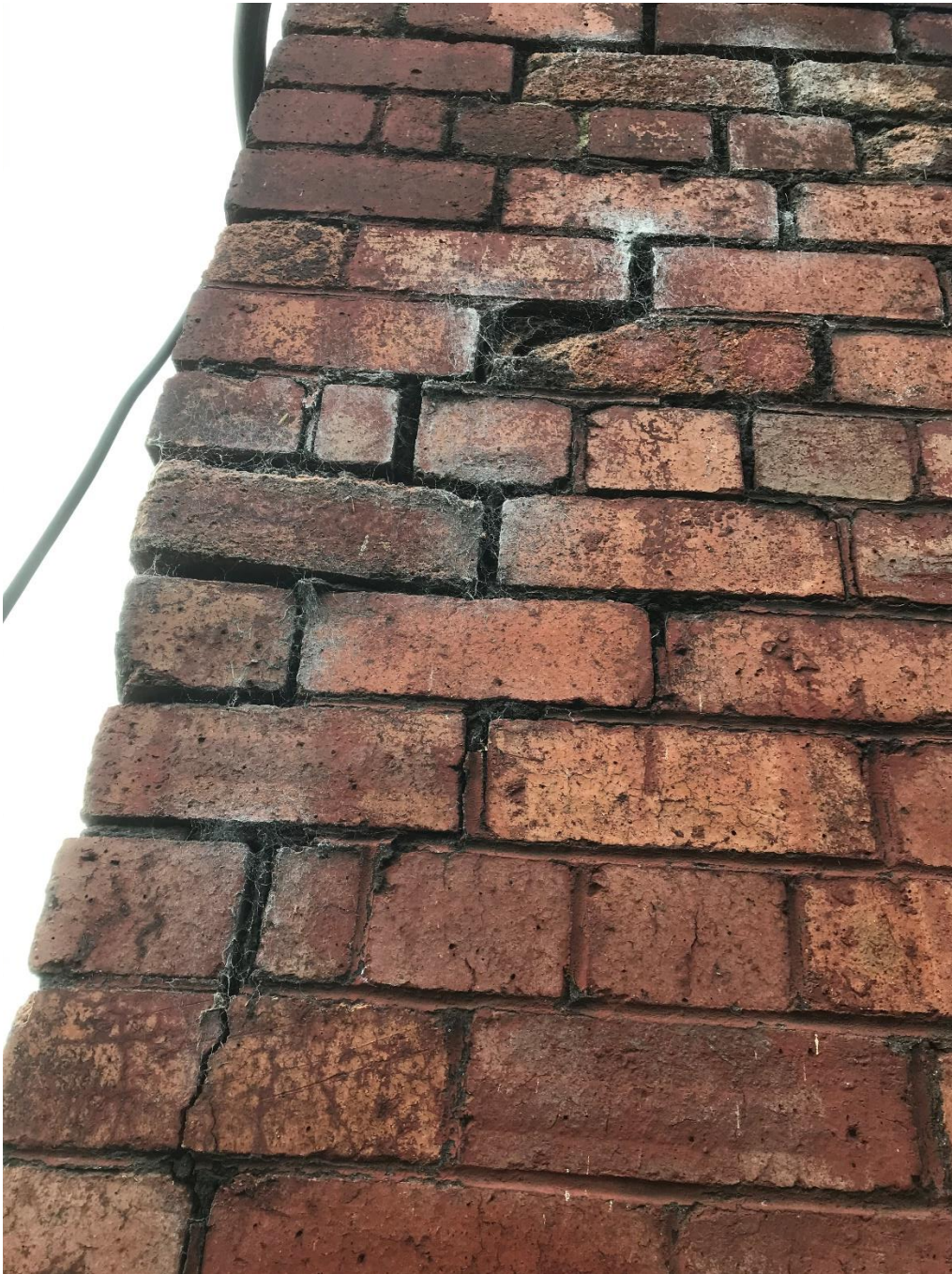
Photograph 17 - South-western corner of Structure B1c, eroded mortar and cracking but covered by cobwebs
