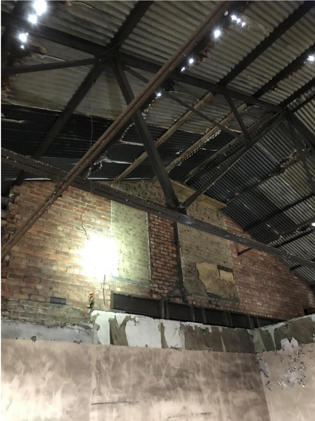
Photograph 12 – Interior of welfare block of structure B1b, note good condition of interior brickwork and intact mortar
