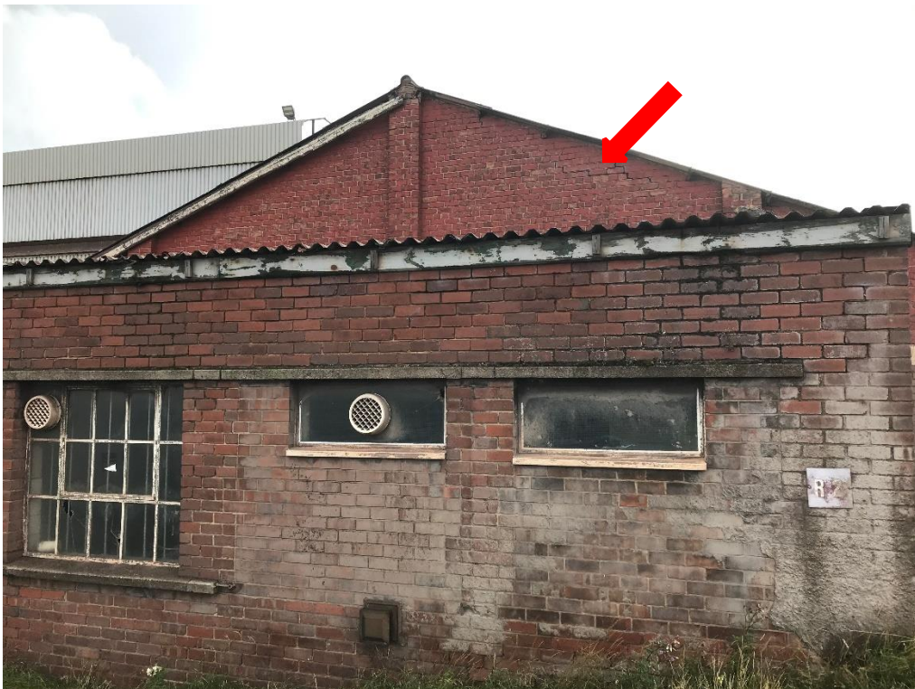
Photograph 14 – Canteen end of structure B1b, note crack in mortar on the gable. Fascia boards on lean-to generally tight against brickwork as per the welfare block.
