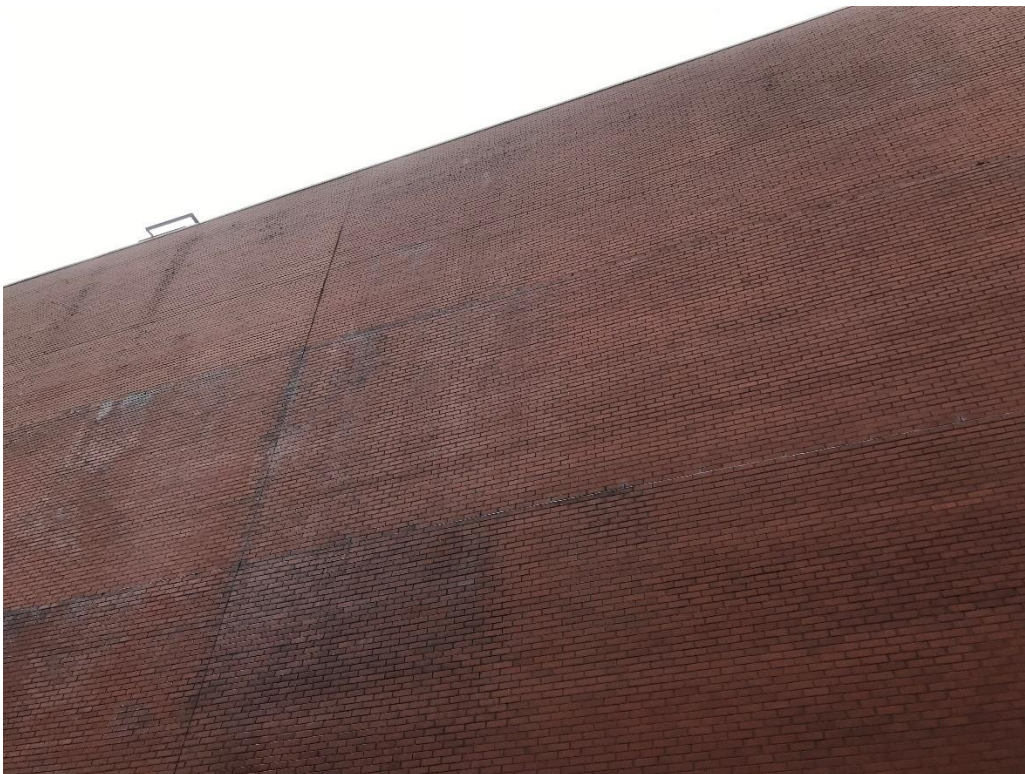
Photograph 24 – View of the brickwork and mortar on north side of Structure B3, no damage
